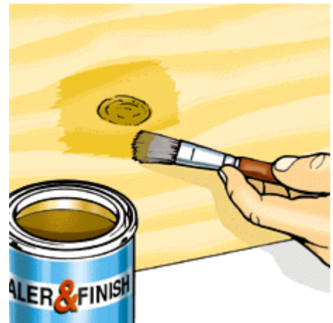
Fig. 12 Apply shellac to any knots before painting. This will seal the knots and prevent sap from bleeding through.
